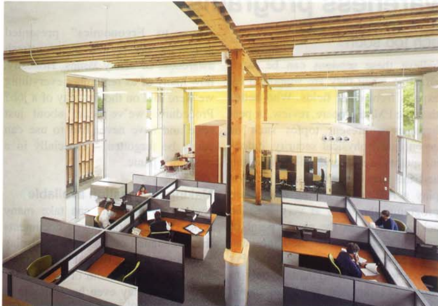
Above: The mezzanine at the east end of the office area overlooks the free-standing meeting room. The base of the column in the central foreground in this view is one of the points at which air enters the building. Fans concealed in the meeting room roof provide additional cooling on the warmest days. Below: The load-bearing, south-facing trellis shades the office and could in time become the outer wall of a greenhouse addition.
